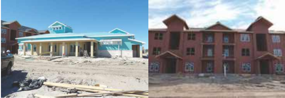
LEASING CENTER (LEFT) AND APARTMENT BUILDING (RIGHT) UNDER CONSTRUCTION
